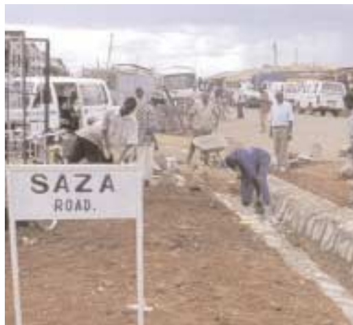
Daventry has worked with Iganga in Uganda to improve its drainage systems, as the area suffers from flash floods
